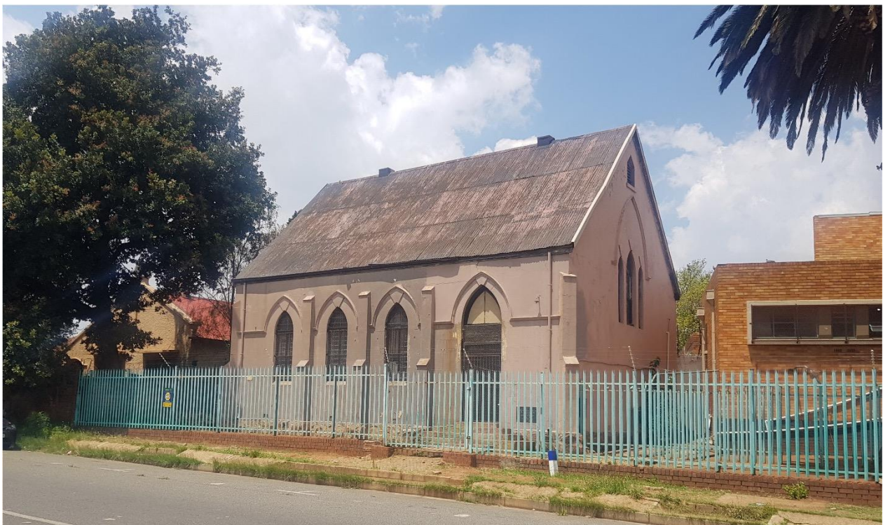
The Roodepoort synagogue left and the Maurice Hockman Talmud Torah and hall adjacent on the right
